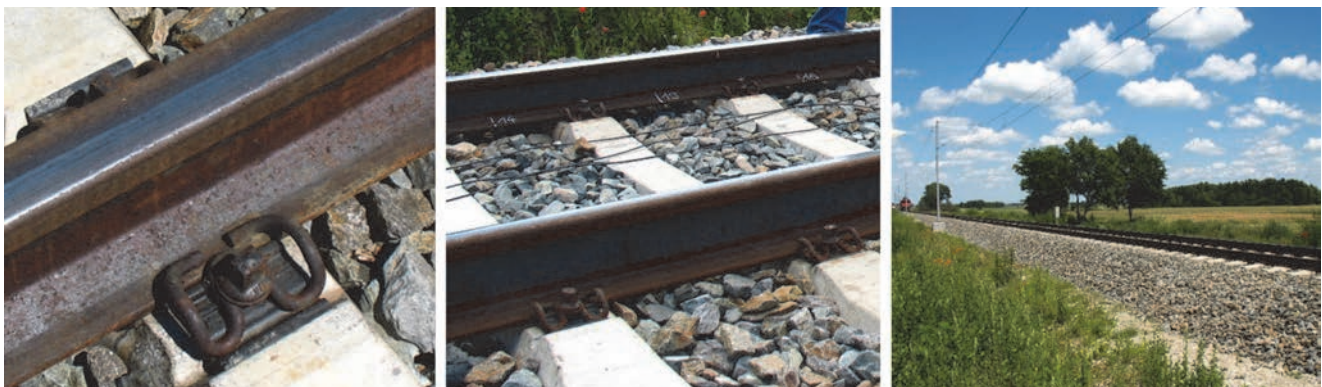
Figure 11. Single track elastic clip SKL-14 (left), sleepers type HŽ – PB85-K (centre) and ballast prism (right)
