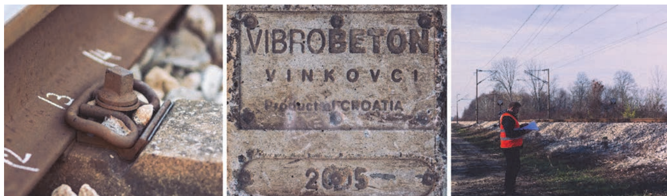
Figure 9. Rail fastened with elastic clip SKL-8 (left side), reinforced concrete sleepers at test section (centre) and ballast prism (right side)
