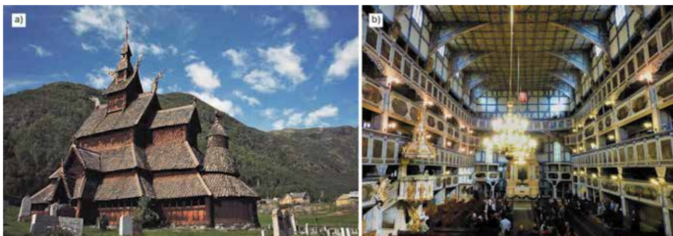
Figure 1. a) Borgund Stave Church (Borgund, Norway) was built sometime between 1180 and 1250 AD (photo by www.wondermondo.com ), b) Interior of Church of Peace (Jawor, Poland) – completed in 1655
