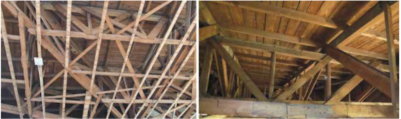
Figure 7. Ceiling of the southern roof of the museum
