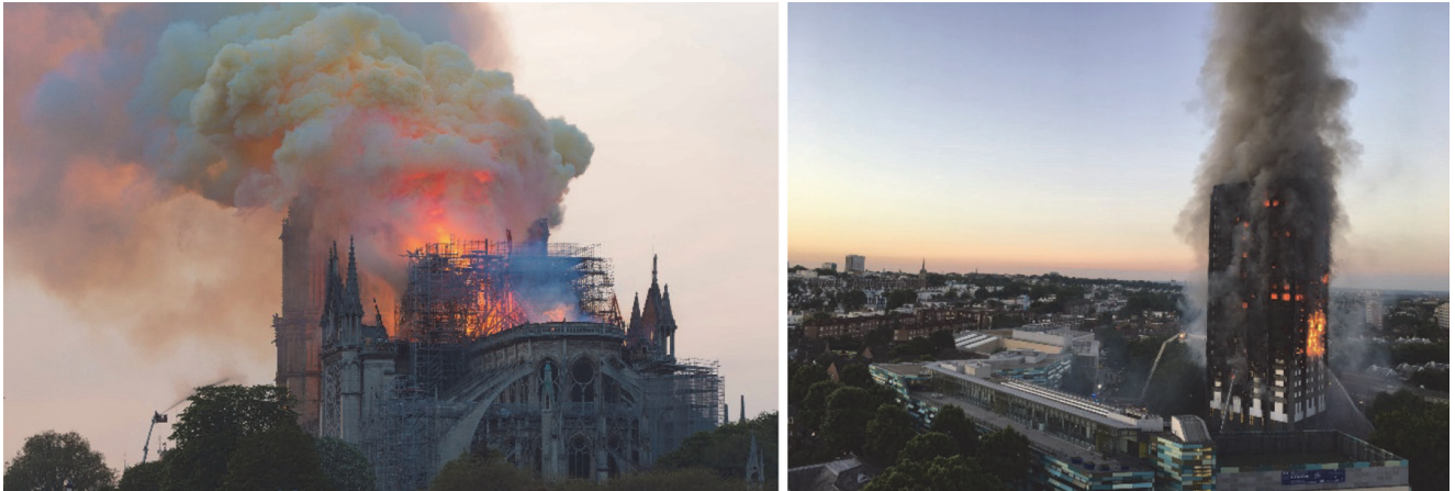
Figure 2. Notre Dame on fire [6], Grenfell Tower on fire [7]
