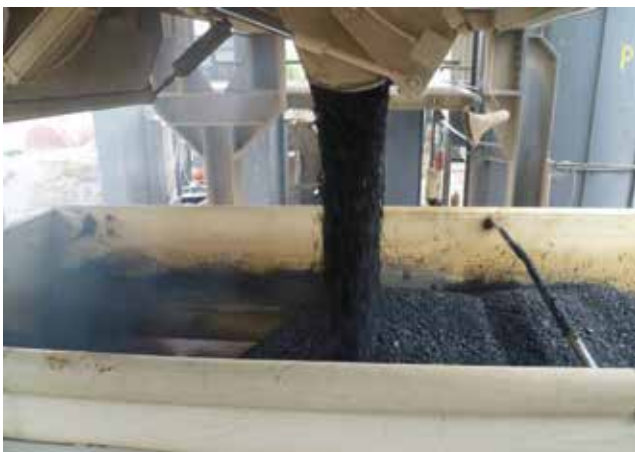
Figure 6. Trial production of asphalt mix with 10% of recycled asphalt
